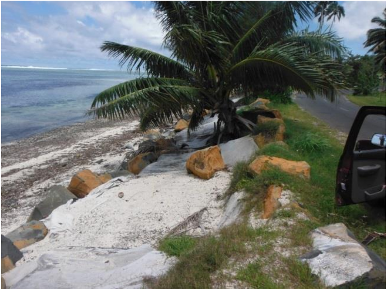
Rock wall outside of the Sheraton/Mirage Hotel site
