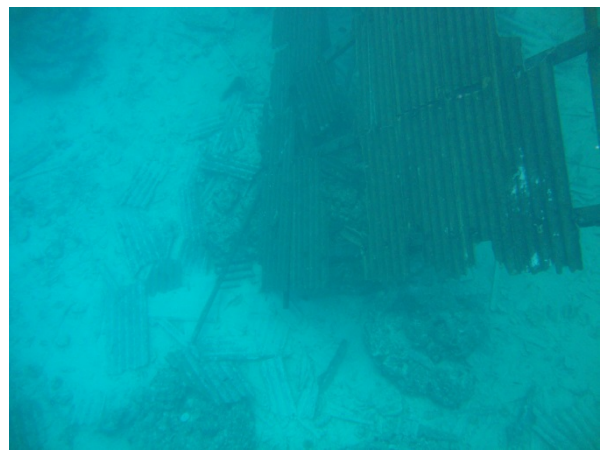
Photo 15: Super six asbestos sheeting from collapsed sorting platform on kaoa.
